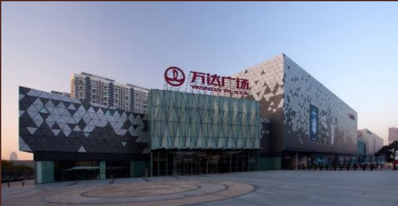
▲ 宁波万达商业综合体立面改造 NINGBO WANDA RETAIL COMPLEX FACADE 中国宁波 Ningbo, China (2011-2012)
